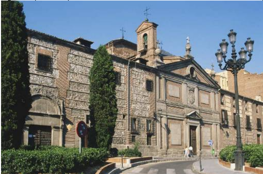
Image 2: (this is the same building but a different picture) http://www.dkimages.com/discover/previews/874/50098422.JPG
